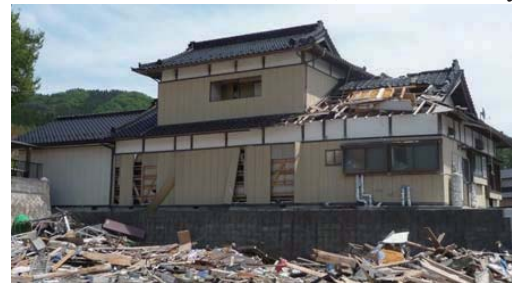
Photo 7.4-30. Wood house (6) which was not carried away in spite of damage on 1 st floor roof system in Akasaki-cho, Oofunato city.
