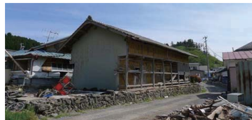
Photo 7.4-32. Survived soil warehouse (10) which seemed to have comparatively slight structural specifications in Akasaki-cho, Oofunato city.
