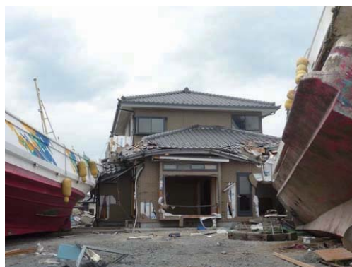
Photo 7.4-26. Wood house remained in spite of ships' crashing in the west of Arahama port.
