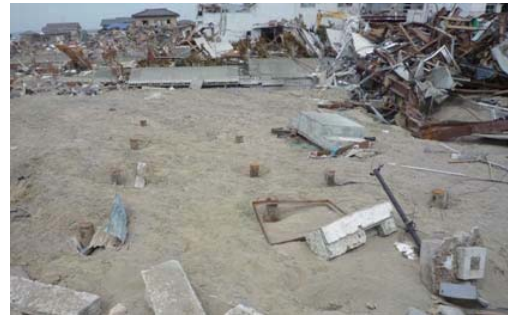
Photo 7.4-11. Steel tube pile left at the original position ([2]) of house in photo 7.4-10.
