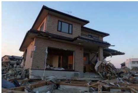
Photo 7.4-10. Wood house ([1]) that was carried away with the base in Yuriage, Natori city.
