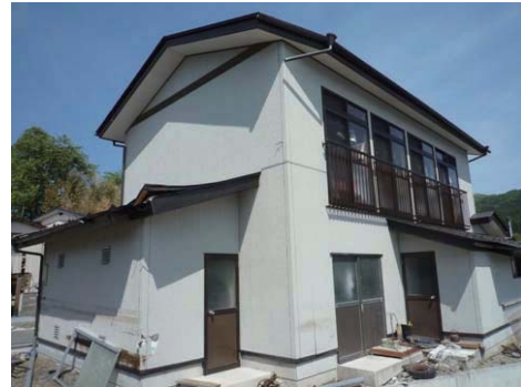
Photo 7.4-28. Wood house (3) without damage under the water depth of over 7 m in Akasaki-cho, Oofunato city.
