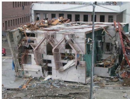
Photo 7.2-9 Overturning of a 3-story steel building
