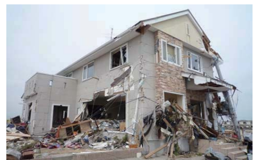
Photo 7.4-19. Light frame construction wood house (12) remained alone
