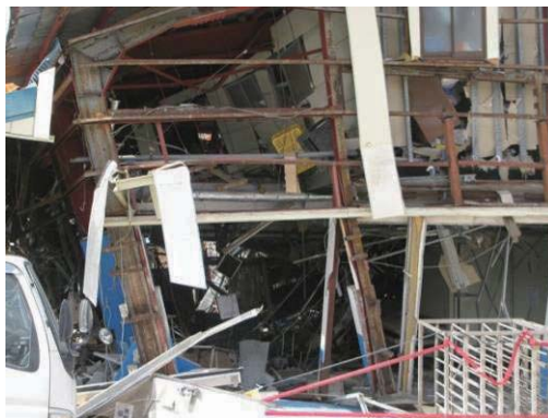
Photo 7.2-11 Tilted gabled roof frame
