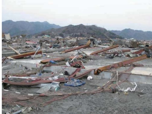
Photo 7.2-8 First-floor columns falling in the same direction
